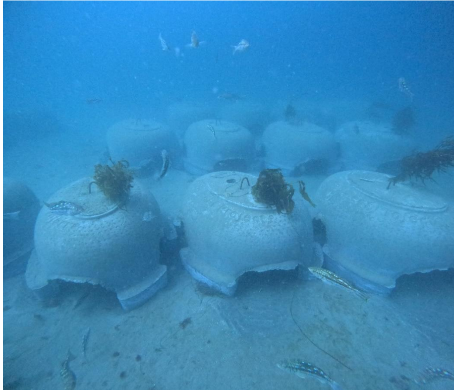
Figure 3. Sandy, flat bottom substrate and newly placed Sea Caves® at Tina Reef.
